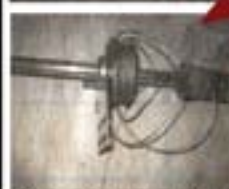
Broken Cables Repaired
